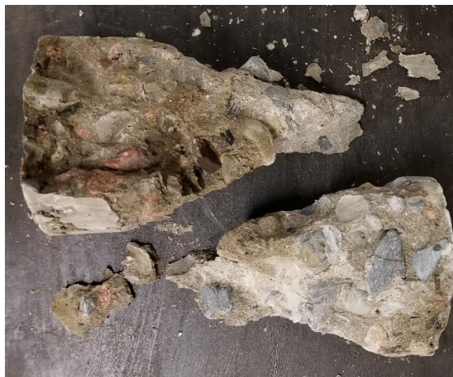
Figure 4.21 Type 1 Fracture Pattern of a Concrete Specimen
