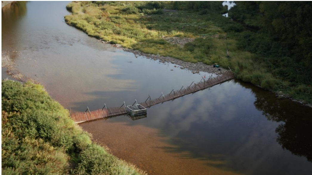
Figure 2. Jacquet River Salmon barrier, NB, Canada. Fish swimming from downriver (upper left corner) are caught in the trap located in the middle, counted, measured, and released on the upstream side of the barrier.
