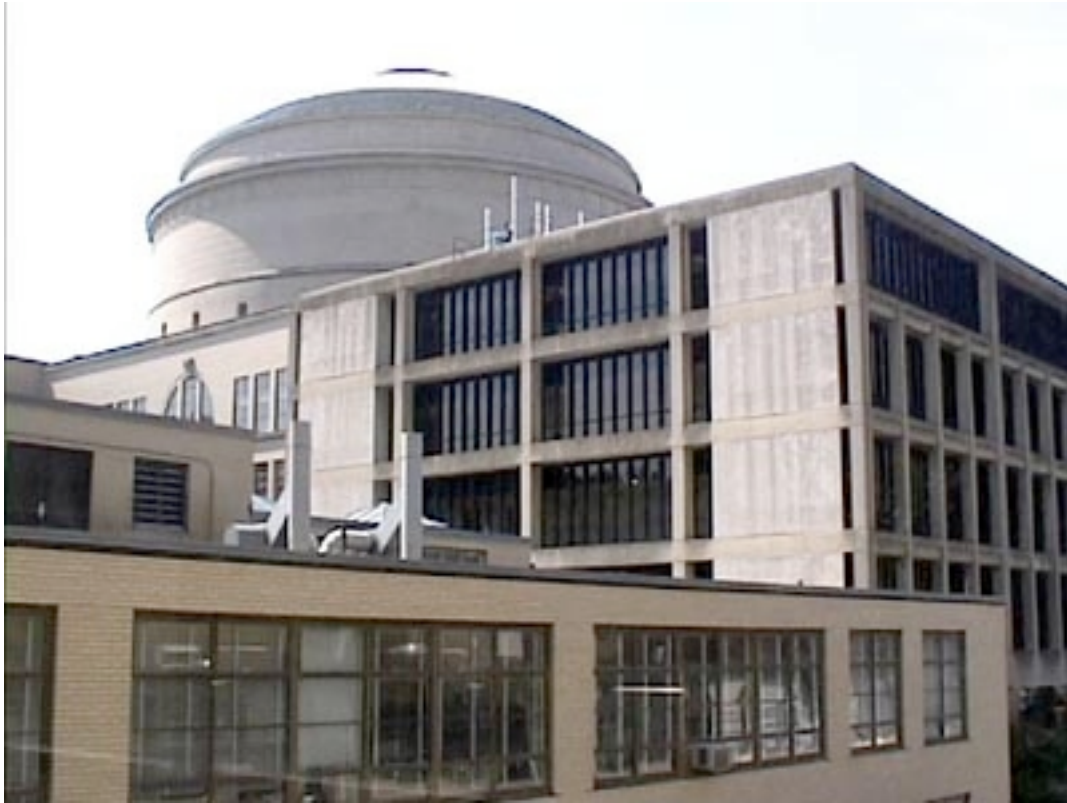
Figure 17: MIT Electrical Engineering Building (Image source: MIT)
