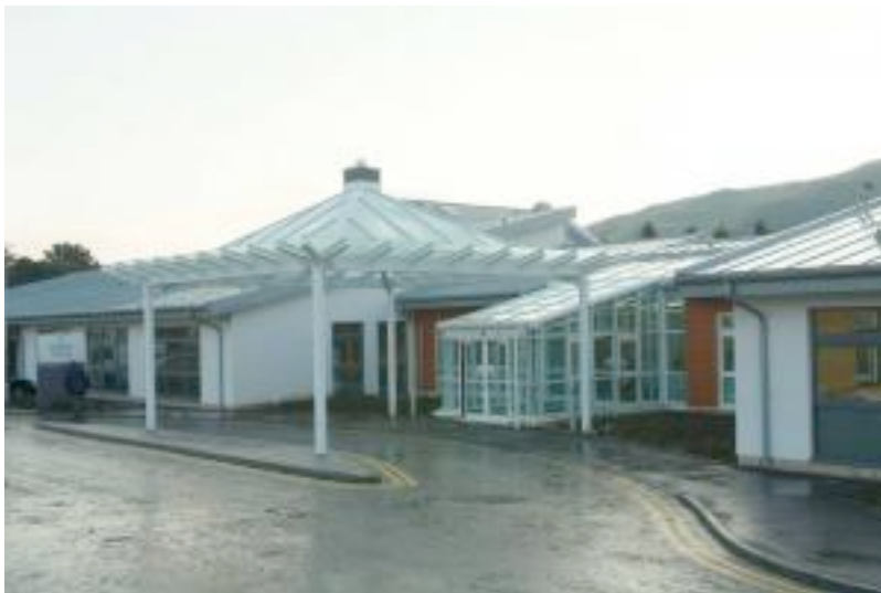
Figure 43: Southeast Mobility and Rehabilitation Technology (SMART) Centre (Image source: NHS)
