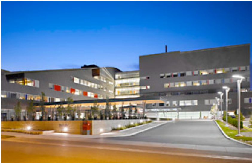
Figure 30: Holland Bloorview Kids Rehabilitation Hospital (Image source: Holland Bloorview)
