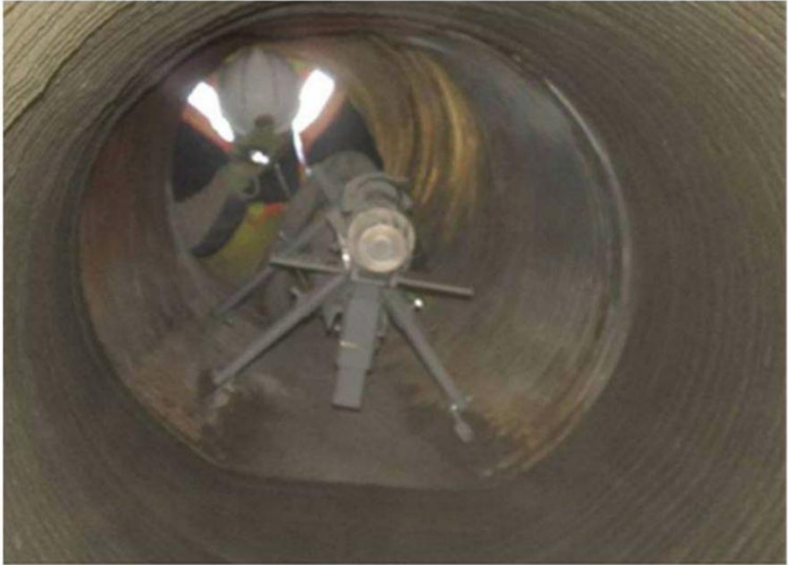
Figure 2.1. Centrifugally Cast Liner Installation [2].
