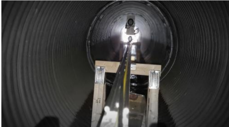
Picture 5. LiDAR mounted to railing system.
