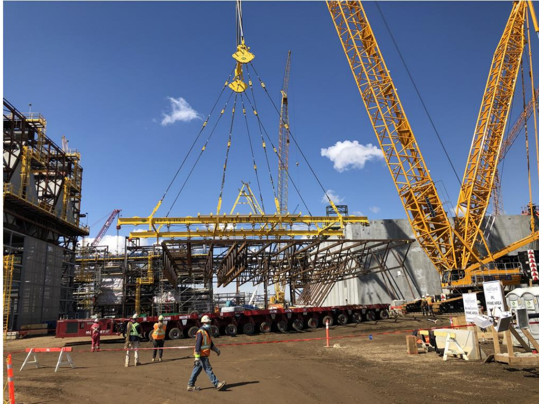
Figure 1: Modular industrial project (photo courtesy of PCL Industrial Management)
