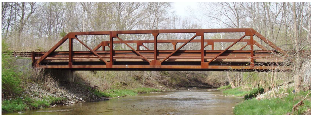
Figure 4 - Load testing of Bridge 251 - Sherman et al. (2020)
