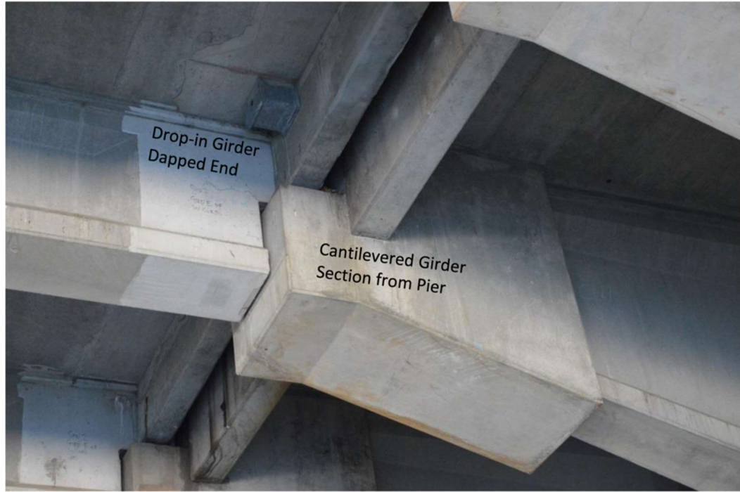
Figure 1 - Dapped end of girder – Zhou and Guzda (2020)
