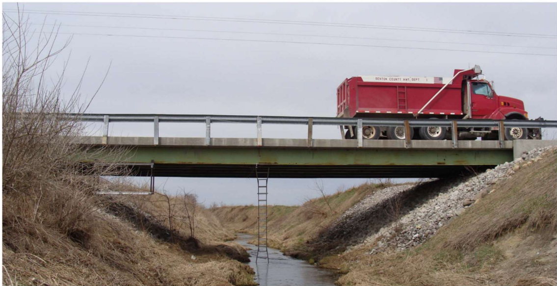
Figure 3 - Load testing of bridge 098 – Sherman et al. (2020)
