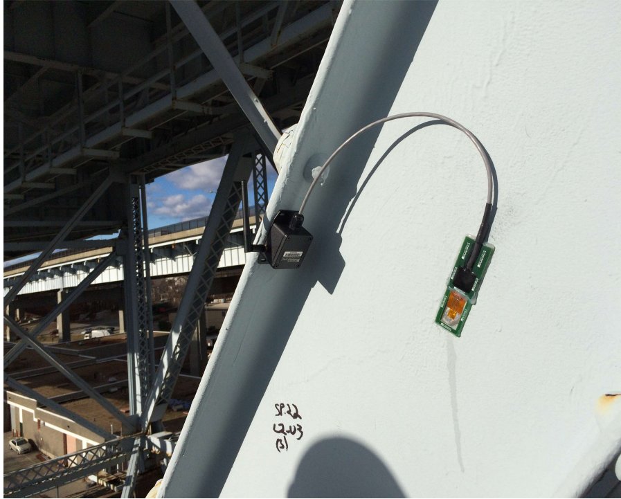
Figure 7 - Typical foil strain gauge installation 2
