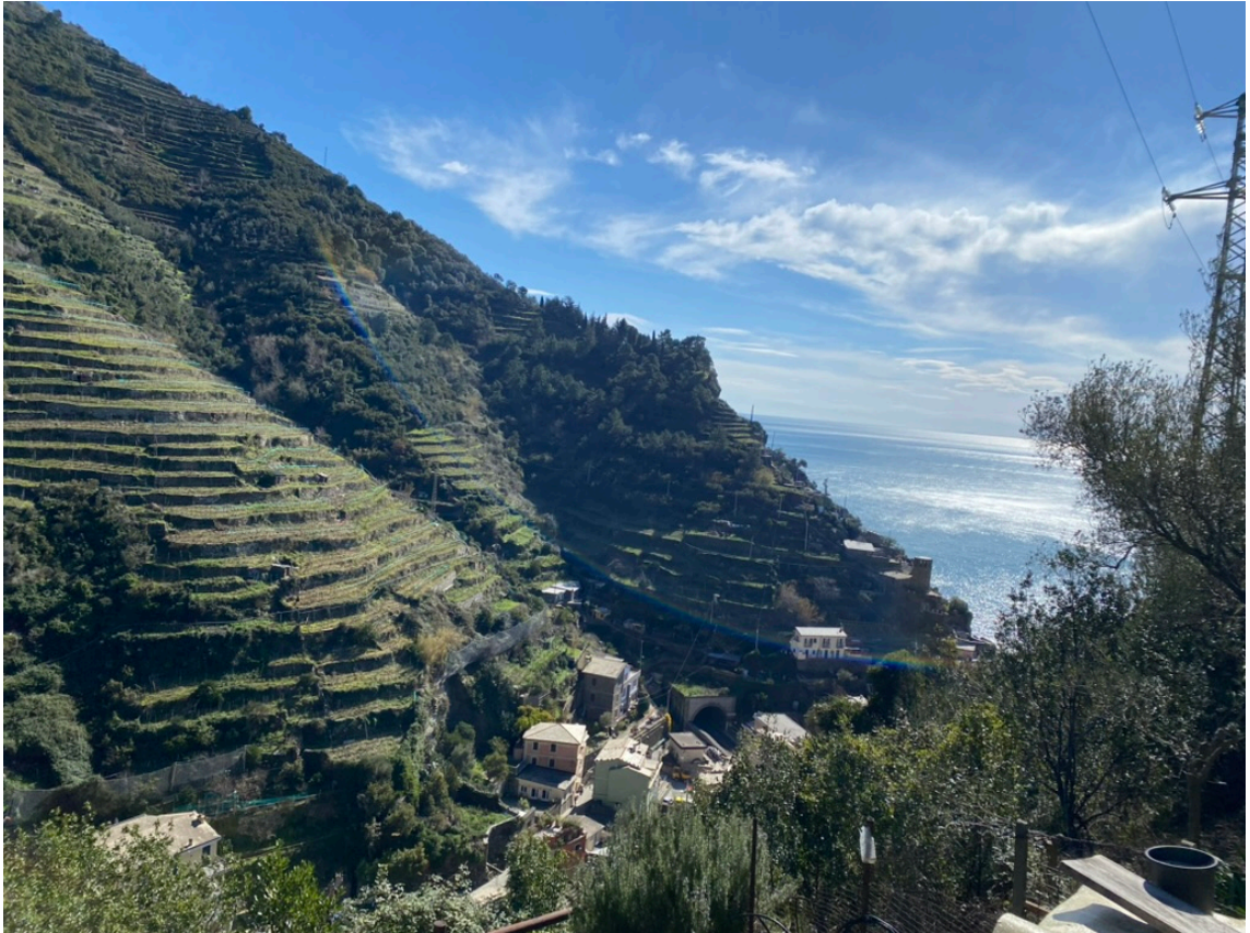
Figure 4: Cinque Terre, a region in northern Italy, is famous for its terraced coast. The inhabitants formed the steep coast to terraces to form narrow gardens. Picture by the author.
