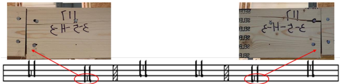
Figure 33 Splitting failure in specimen 3-5-H
