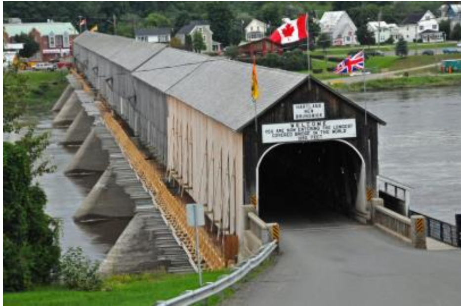
Figure 2 Hartland Covered Bridge
