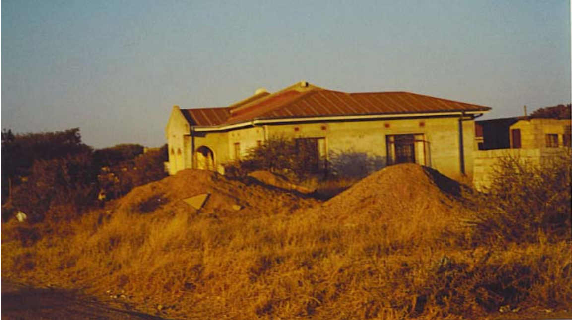
FIGURE I.3: Photograph of recently completed house in Mogoditshane village
