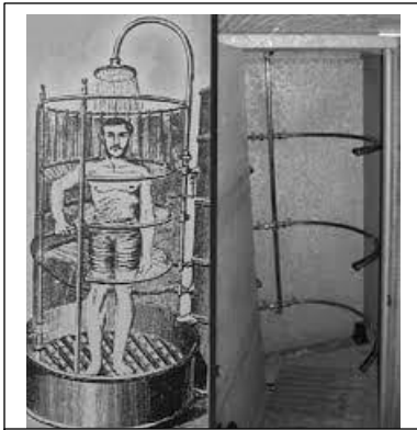
Shower System in Disinfection Building (Parks Canada)
