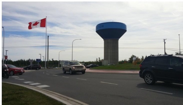
Figure 3.1: Ground level water tower view
