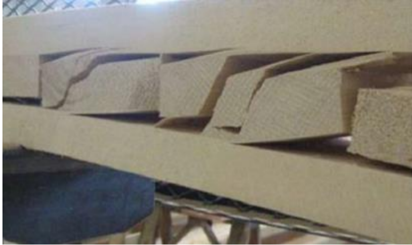
Figure 1.5 The failure of CLT because of rolling shear (Yuan 2016).
