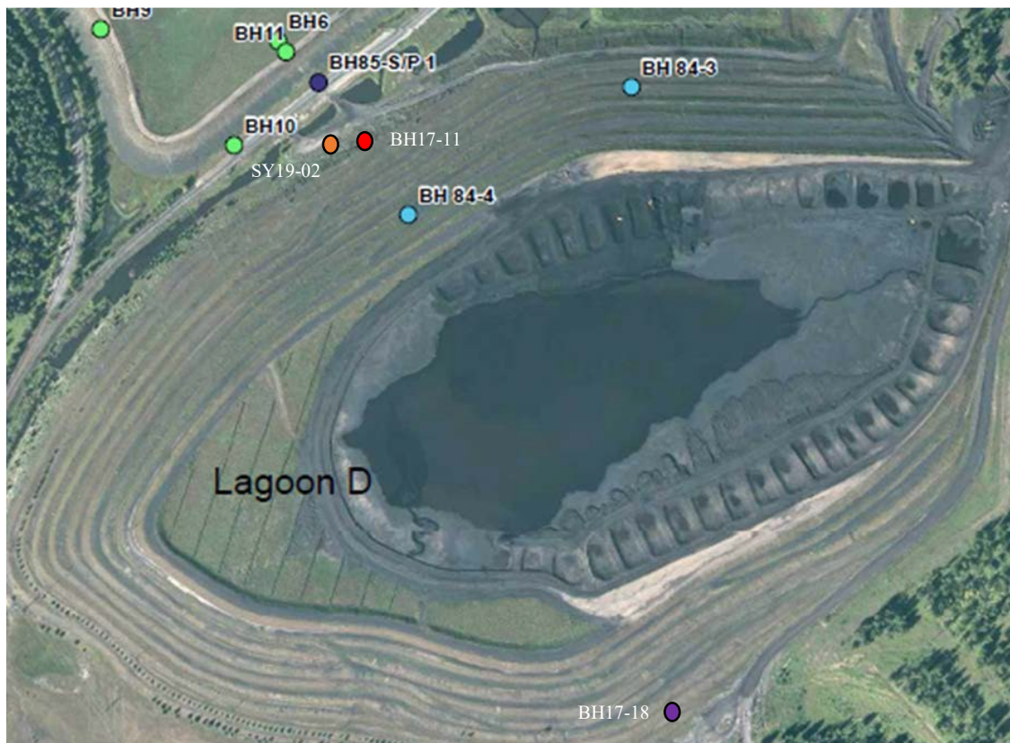
Figure 5.3. Locations of boreholes in Lagoon D
